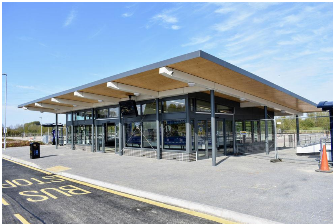
Figure 11.5: New terminal building constructed with the expansion of Seacourt Park and Ride in West Oxford 60
